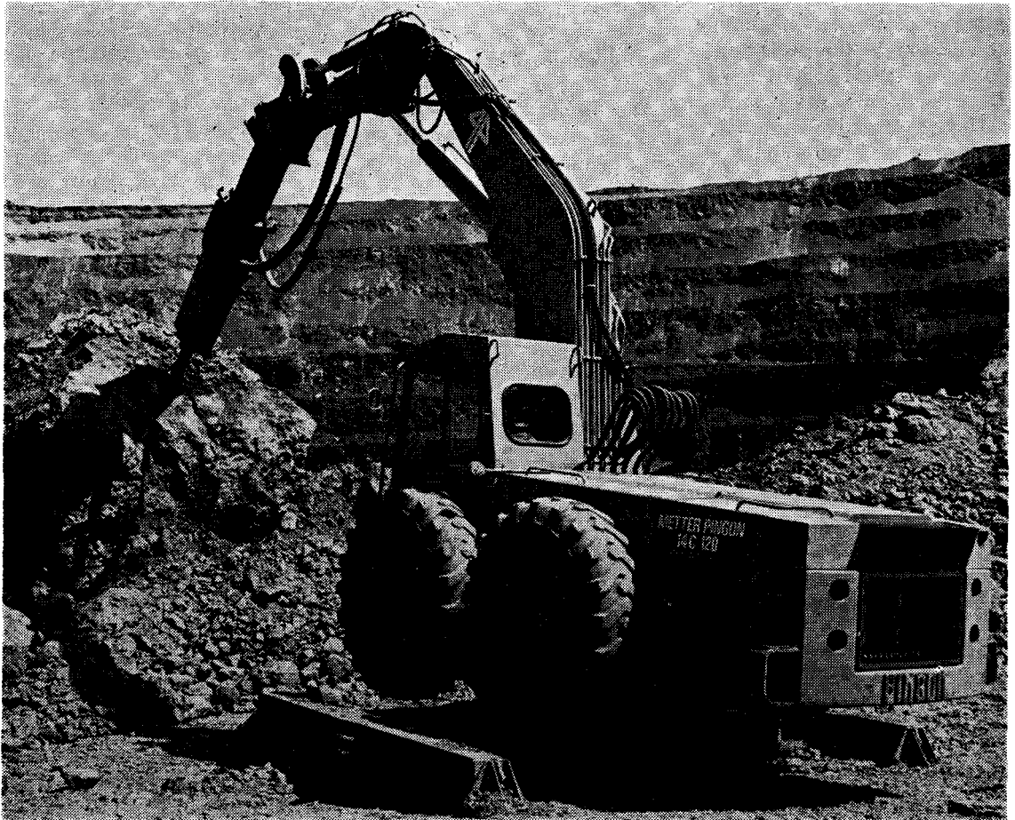
Fig. 24—Hydraulic rock breaker used instead of secondary blasting
