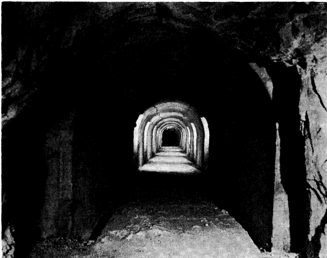
Fig. 12—View of a completed block-cave drift
