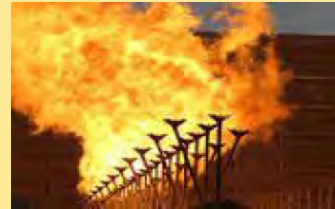
Multipoint ground flare
