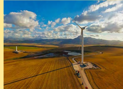
Wind farm, Western Cape
