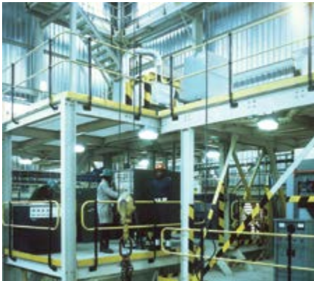
Inside the Aquarium Diamond Recovery Plant at Jwaneng Mine (Debswana, 2009)
