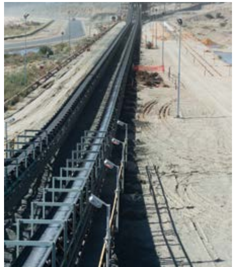
Juanang Cut 8 replacement ore conveyor (Debswana, 2011)
