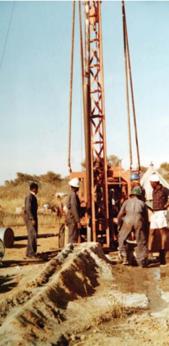
Jumper Drilling a kimberlite prospect in the Kgalagadi District (M. Brook, 1982)
