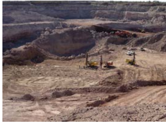
Production blast drilling at B/K11 pit (Firestone Diamonds, 2011)
