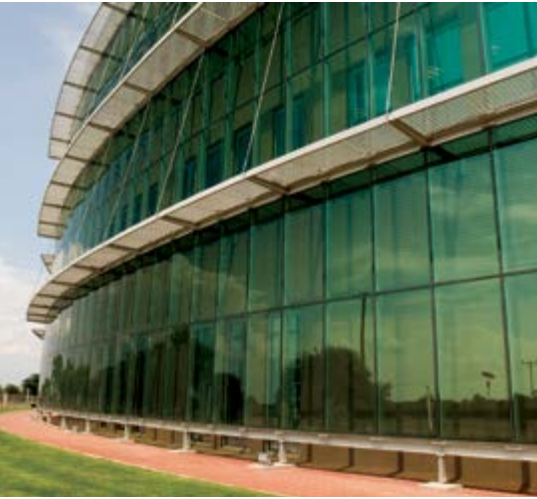
DTCB Sorting Building, Gaborone (DTC, 2008)
