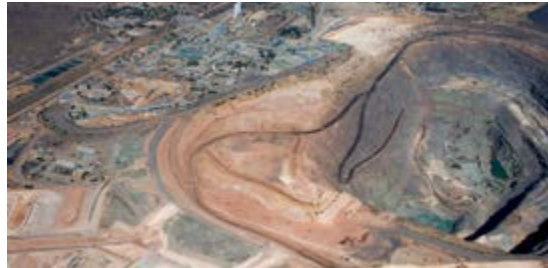
Jwaneng Mine, Cut 8 (Debswana, 2011)
