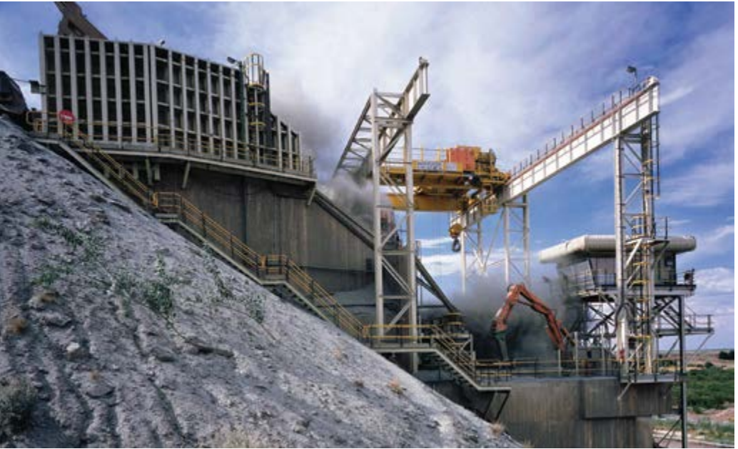
Orapa Mine Primary Crusher (Debswana, 2002)
