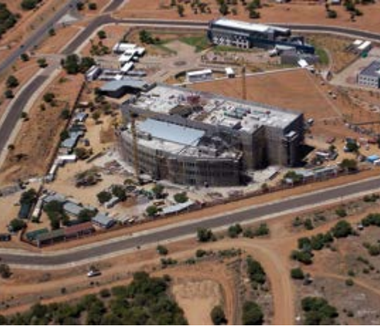
DTCB building under construction (DTCB, Courtesy, Peter McMorran, 2007)
