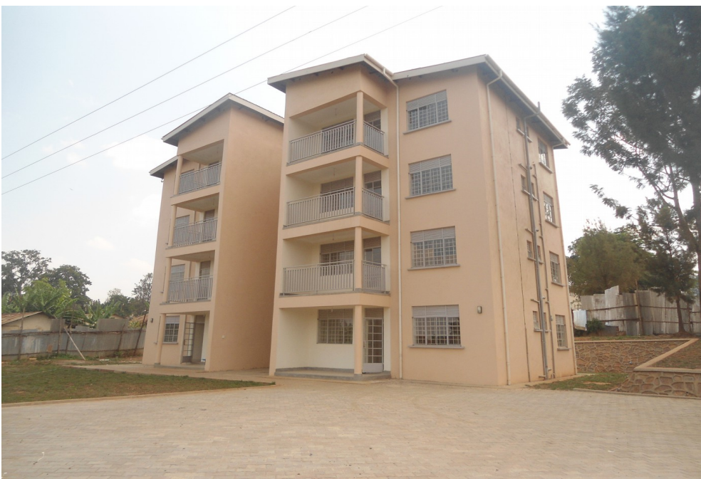
Newly constructed staff Units at Mbarara RRH
