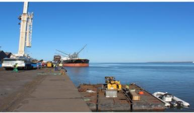
Berths 6, 7 & 8 rehabilitation to deliver 2 deep water berths (draft = 14m & LOA = 250m)
